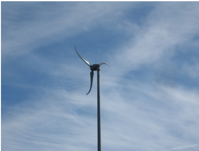
A “small wind” electric system turbine
